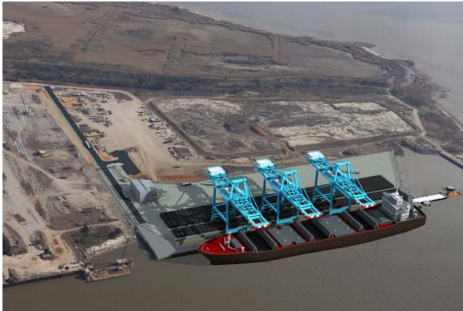
Aerial shot of the new $115 million Pinto Terminal in Mobile, Alabama with computer-generated cranes and ship showing the facility's future capabilities. (high-res file available)
